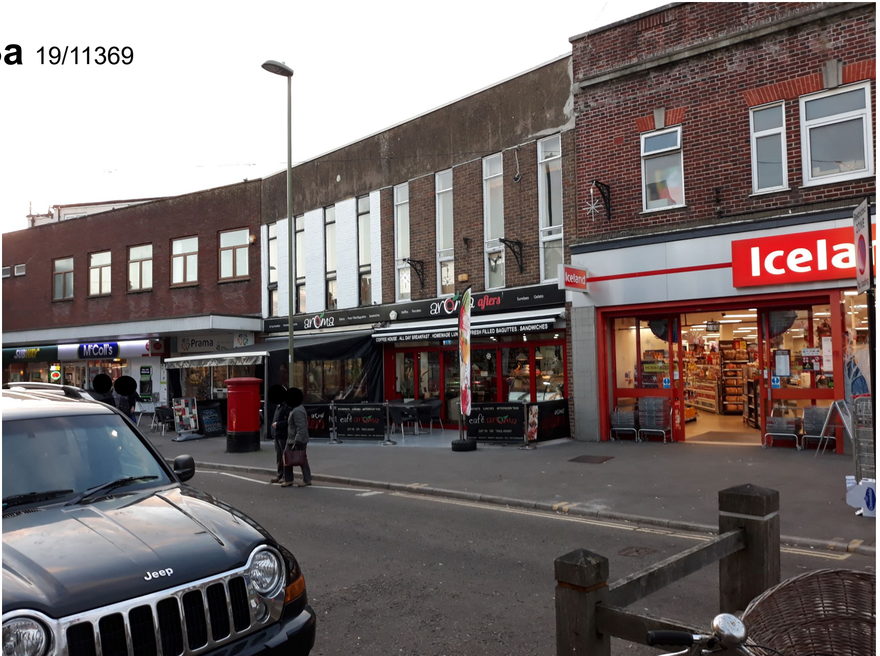
7 Wider street view
